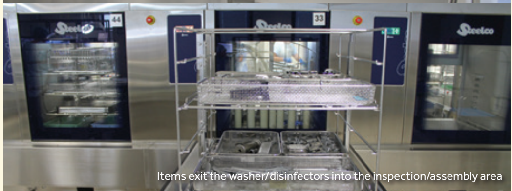
Andy Gella loads items onto conveyor, the fully automated system will then assign the cart to the next available washer/disinfectors
